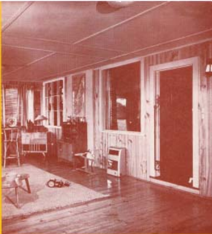
The Radiata Pine shown above has finished but untreated, but treated use of this timber is with floor coverings.
